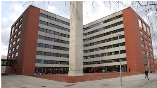
Figure 1.2: The FIT building.
